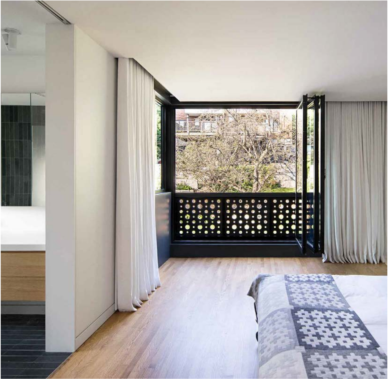
In the main bedroom, large concertina doors open up to the rear garden. A perforated balustrade affords privacy.
