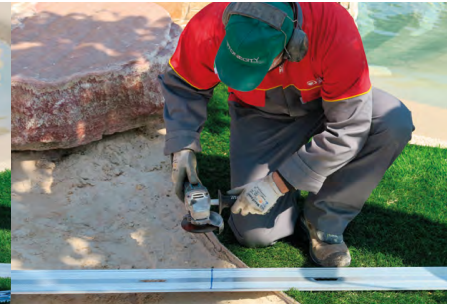
3. Taglio a misura con flessibile. 3. Cutting to size with flexible saw.
